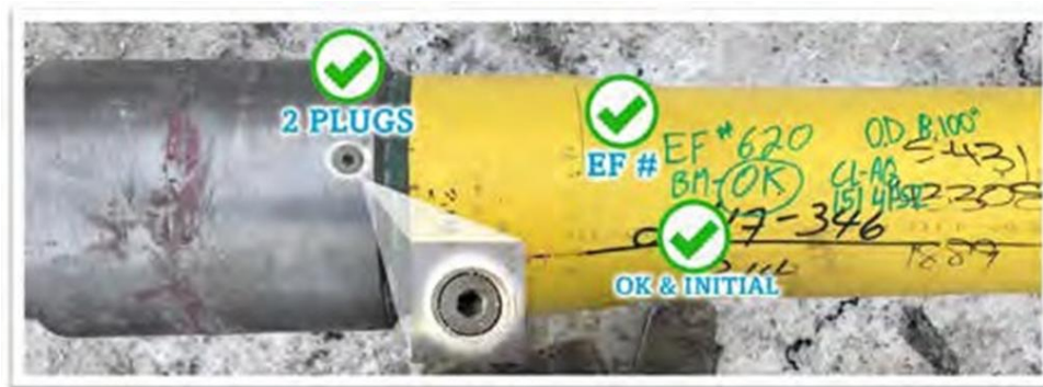
Completed ClickWeld® ready for coating
