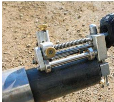
Scrape the poly to proper OD
