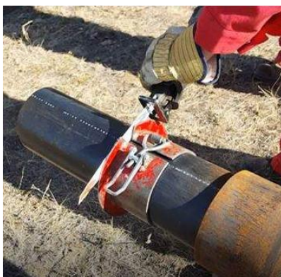
Cut the liner to length
