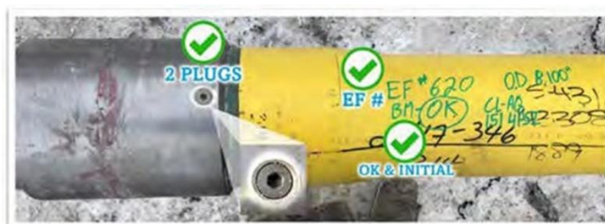
Completed ClickWeld® ready for coating
